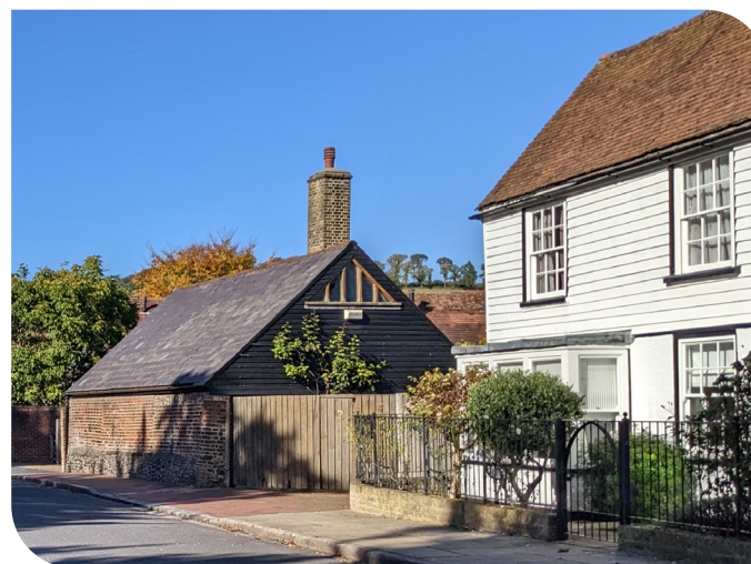
Weatherboarding is sometimes used to clad houses, and usually then painted a pale shade; more often it is employed to clad ancillary or farm buildings, when it is traditionally tarred black if softwood is used
