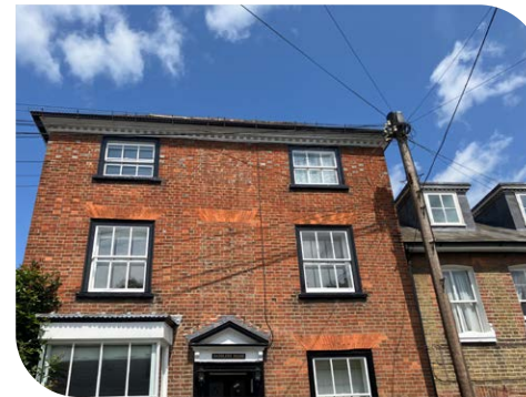
Sash windows and panelled timber door
