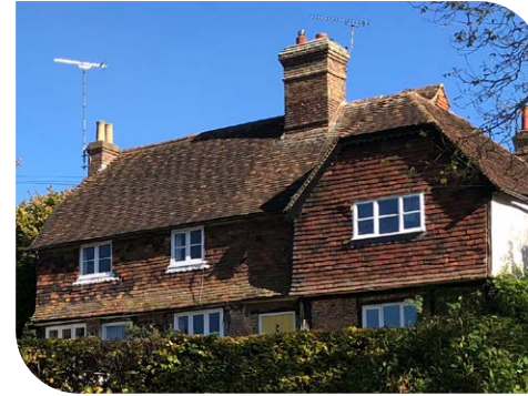
Clay tile hanging
