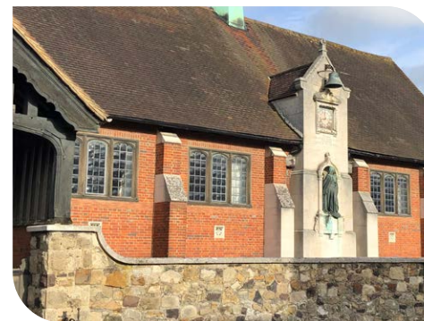
Timber casement windows with leaded lights
