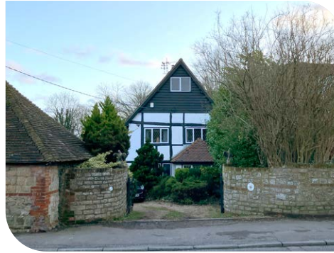
Timber framed buildings
