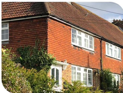
Clay tile hanging
