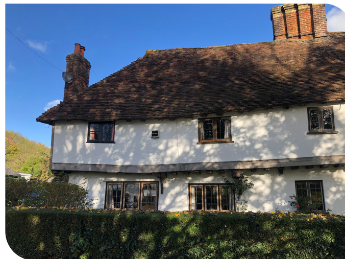
Lime render has been applied to buildings for centuries, in this case to a timber-framed house
