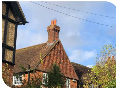
Tall brick chimneys
