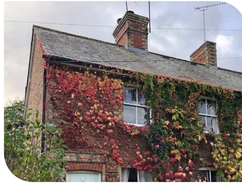
Welsh slate roofs
