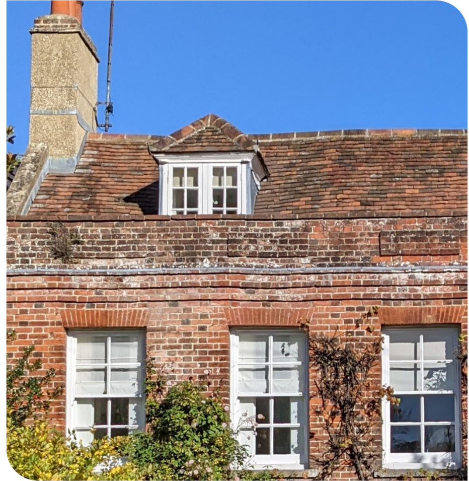
Kentish 'peg tiles', irregular roof line and dormer window. Traditionally, where they are used, dormer windows are small and visually subservient
