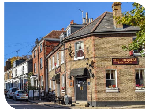
Welsh slate roofs
