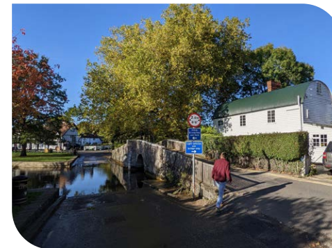
Old mill buildings
