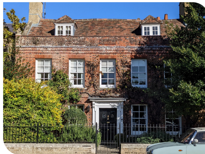
Handmade brick, with flush lime pointing
