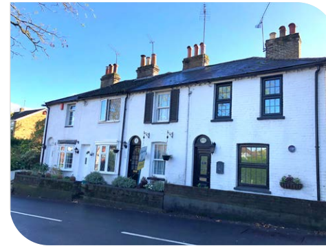
Welsh slate roofs
