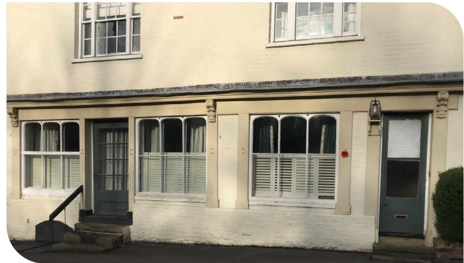
Historic shopfront, carefully retained
